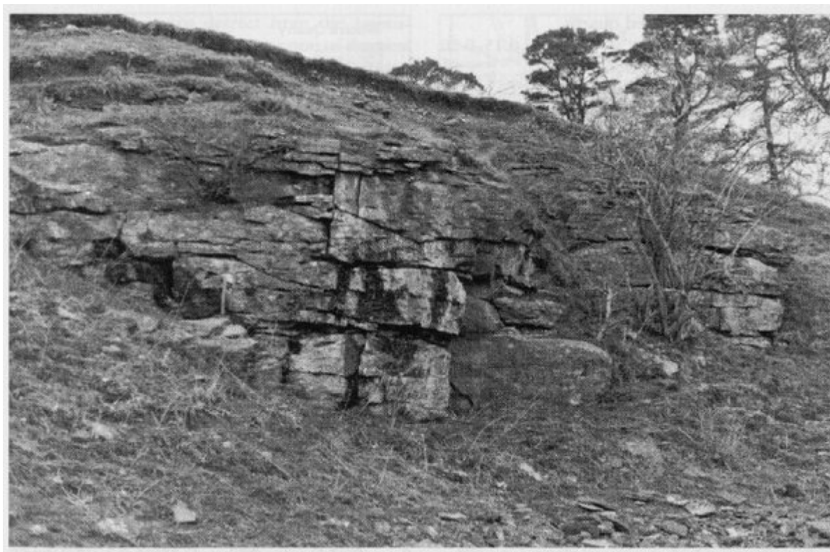
(Figure 4.18) View of the eastern quarry at Hackness Head, showing the massive, bioclastic limestones of Subdivision 2 overlain by coral rubble (Subdivision 3) just below the grass at the top. Hammer shaft (mid-left of picture) is 30 cm. (Photo: J.K. Wright.)
