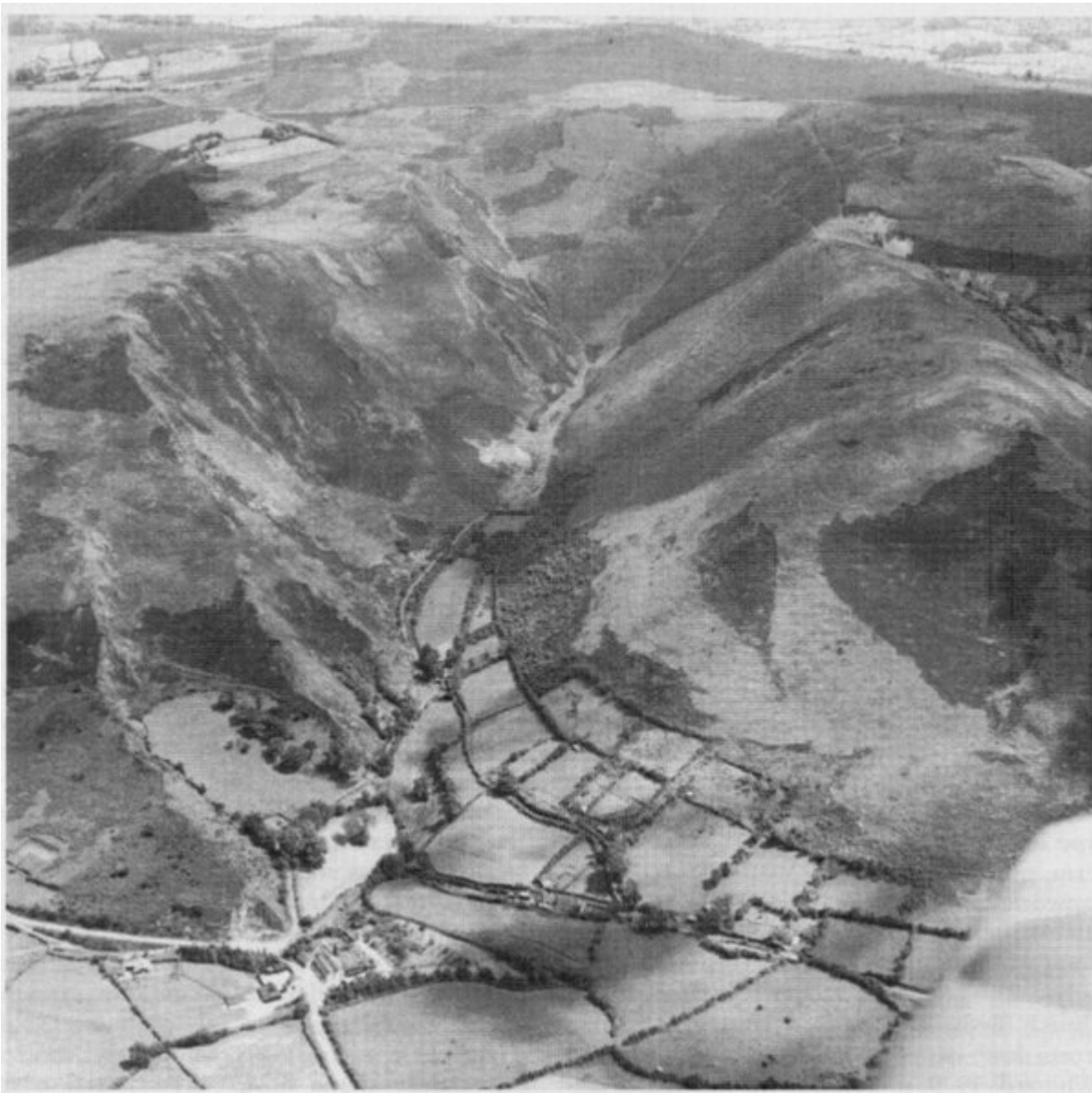
(Figure 10.3) View eastwards along Mytton Dingle. The Mytton Flags Formation, cropping out on the north side of the valley, dips steeply towards the viewer and strikes obliquely south-west. The ridge on the left is Blakemoorflat; Green Hill, on the right, slopes down into Perkins Beach. (Photo: Cambridge University Collection of Air Photographs, BM 13: copyright reserved.)
