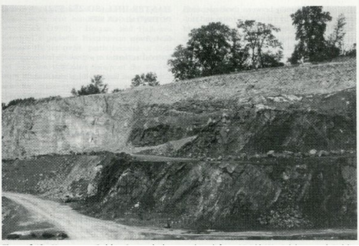
(Figure 5.19) View across Dolyhir Quarry, looking northward from [SO 244 583]. Sub-horizontal Dolyhir Limestone overlies westward-dipping Longmyndian strata of the Yat Wood Formation. Both units are displaced across a west-dipping dip-slip normal fault. (Photo: N.H. Woodcock.)
