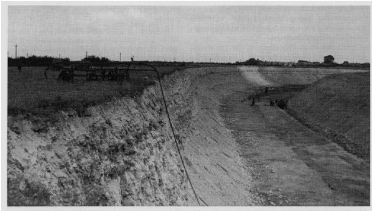
(Figure 4.17) Irchester Old Lodge Pit; general view of former ironstone pit showing bared bed of ironstone (Northampton Sand Formation) and overburden of Grantham, Rutland and Blisworth Limestone formations. (Photo: British Geological Survey, No. A8194, 1945.)
