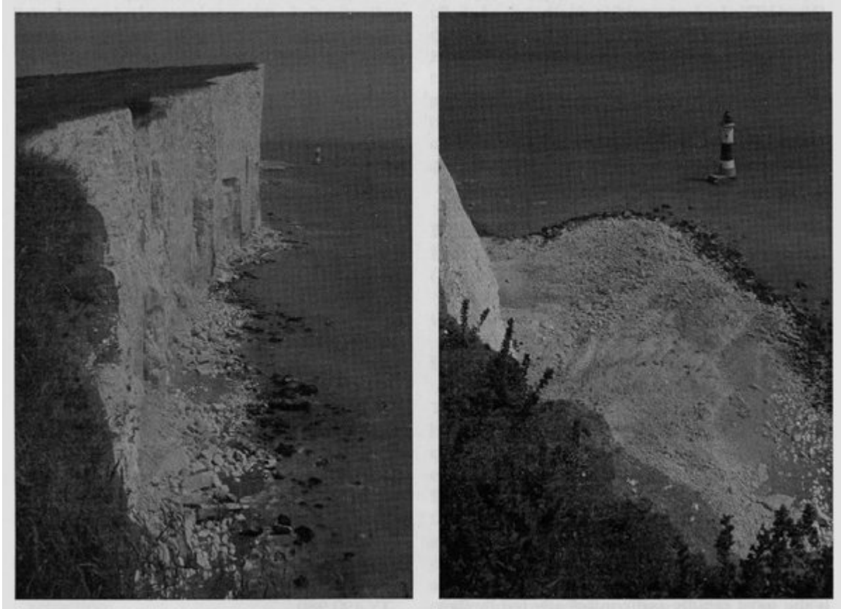
(Figure 4.26) (a) Beachy Head, cliff top view looking east, the cliffs are characterized by slab failures in the lower cliff that gradually undermine the upper cliff. (b) Cliff collapse at Beachy Head, early 1999; the failure affected the whole cliff face and produced a very large debris area at the cliff foot. (Photos: V.J. May.)
