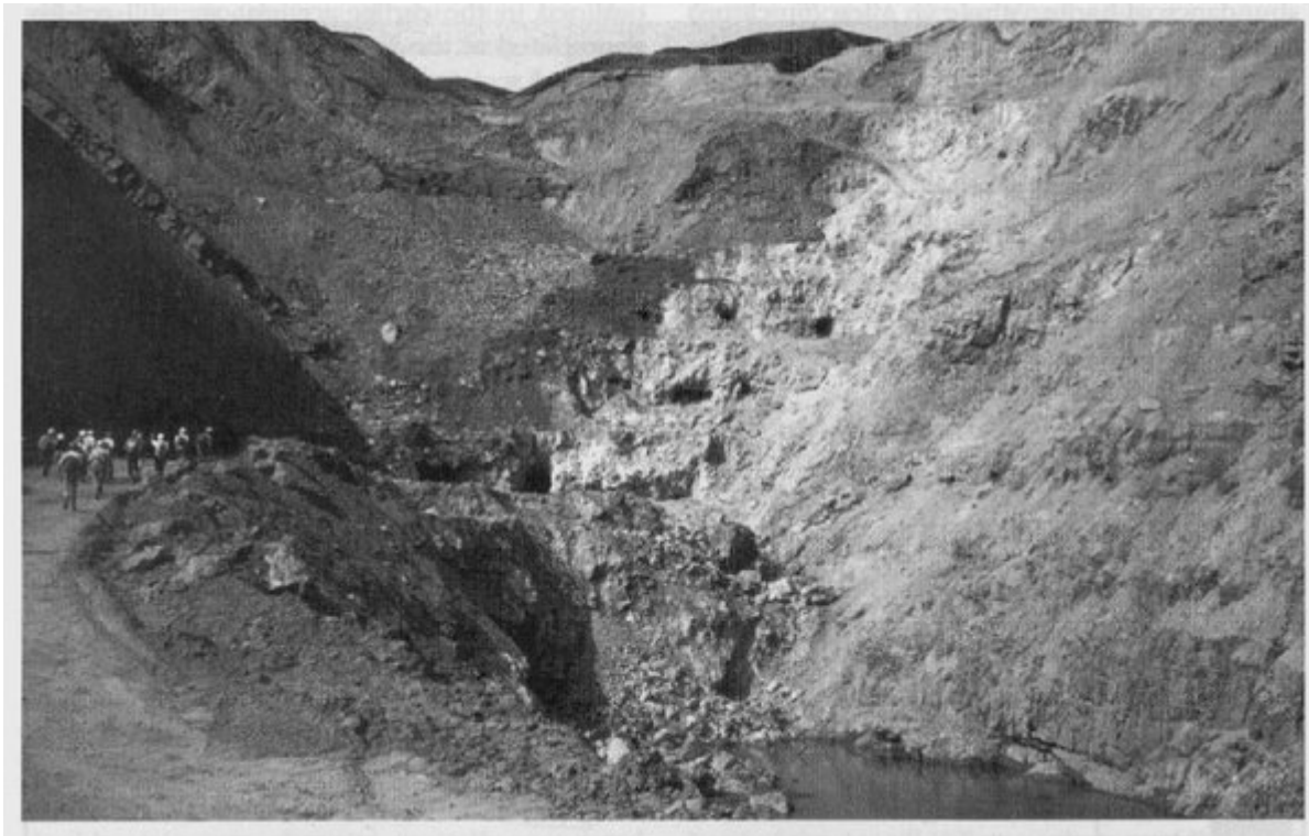
(Figure 3.15) View of main opencast workings at Closehouse Mine, in 1984, showing the wide barite orebody in which old levels from previous underground workings may be seen. Almost horizontal limestones and shales on the footwall are exposed on the right of the picture. Steeply folded sandstones and limestones on the hangingwall can be seen on the left. (Photo: B. Young.)
