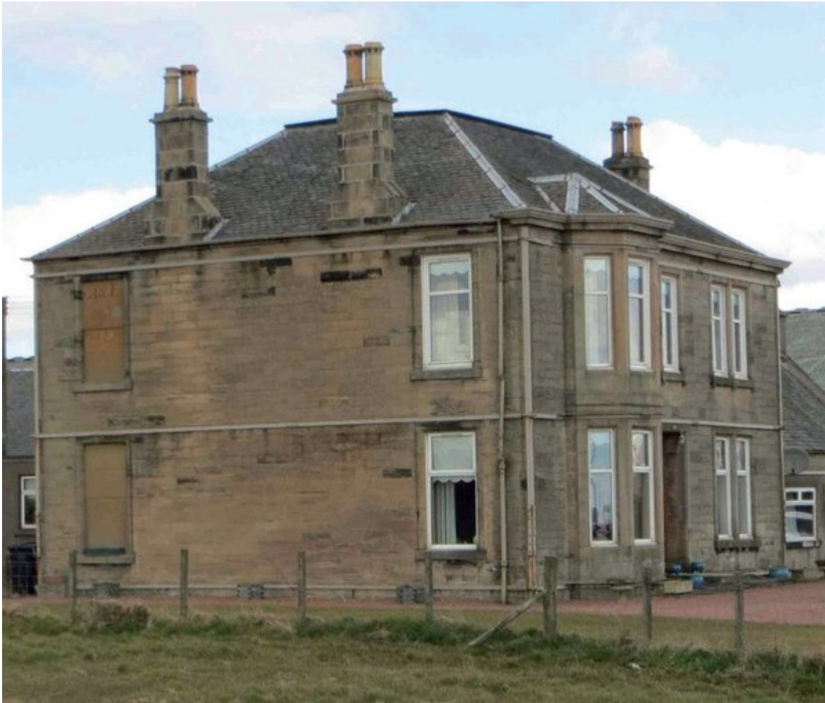
(Plate 3.3) Locality 3.4. Evidence of ground instability due to shallow coal workings; house with restraining horizontal and vertical metal straps, near Bellsdyke roundabout.
