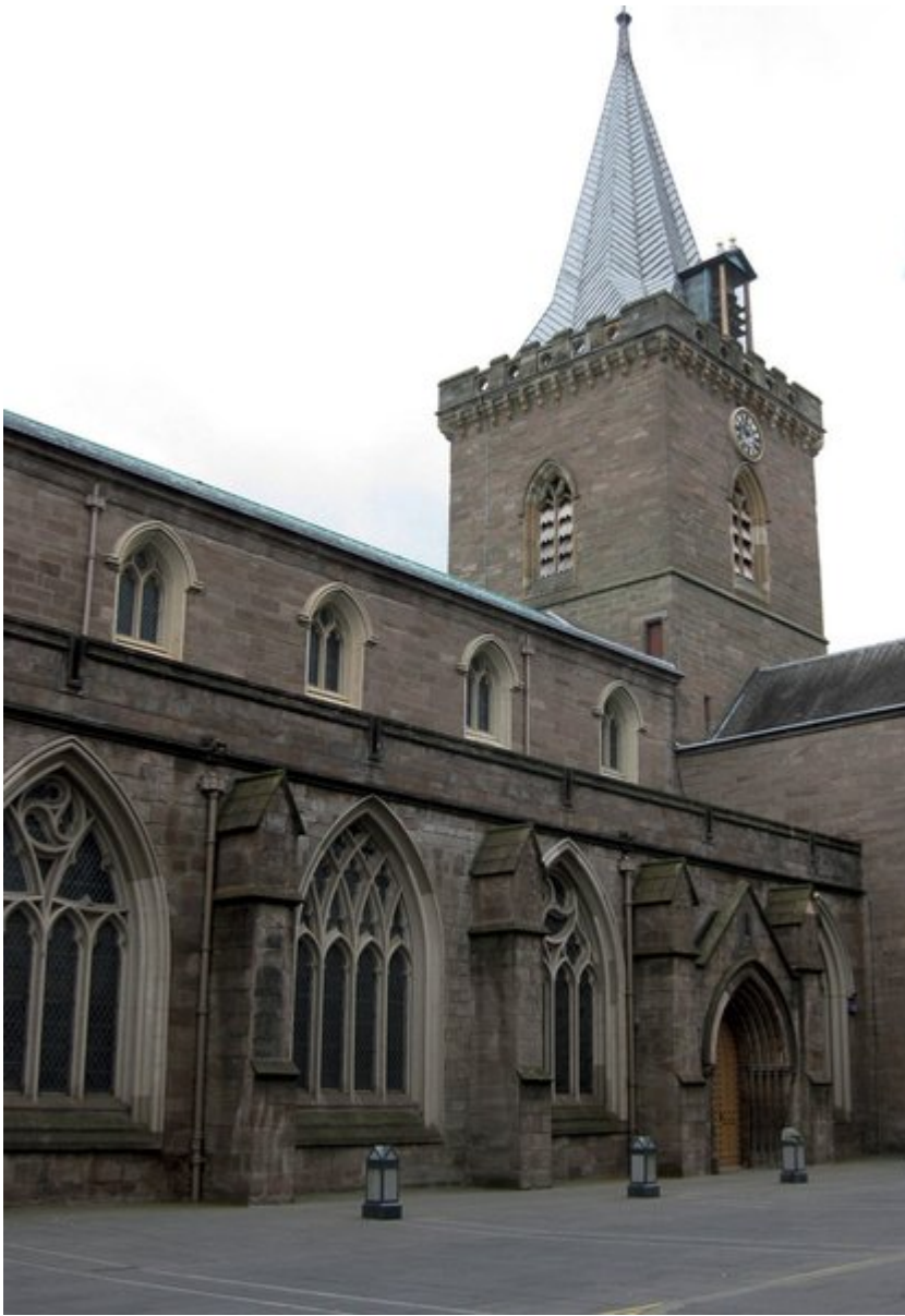
(Plate 16.1) Locality 16.1. St John's Kirk; sandstones from various quarries in Scone Sandstone Formation.
