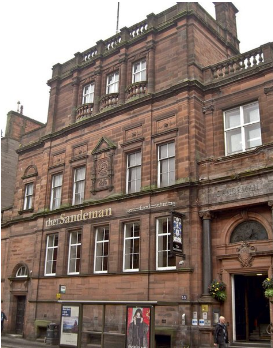
(Plate 16.5) Locality 16.13 Sandeman Building; red Permian sandstone, Locharbriggs, Dumfries.
