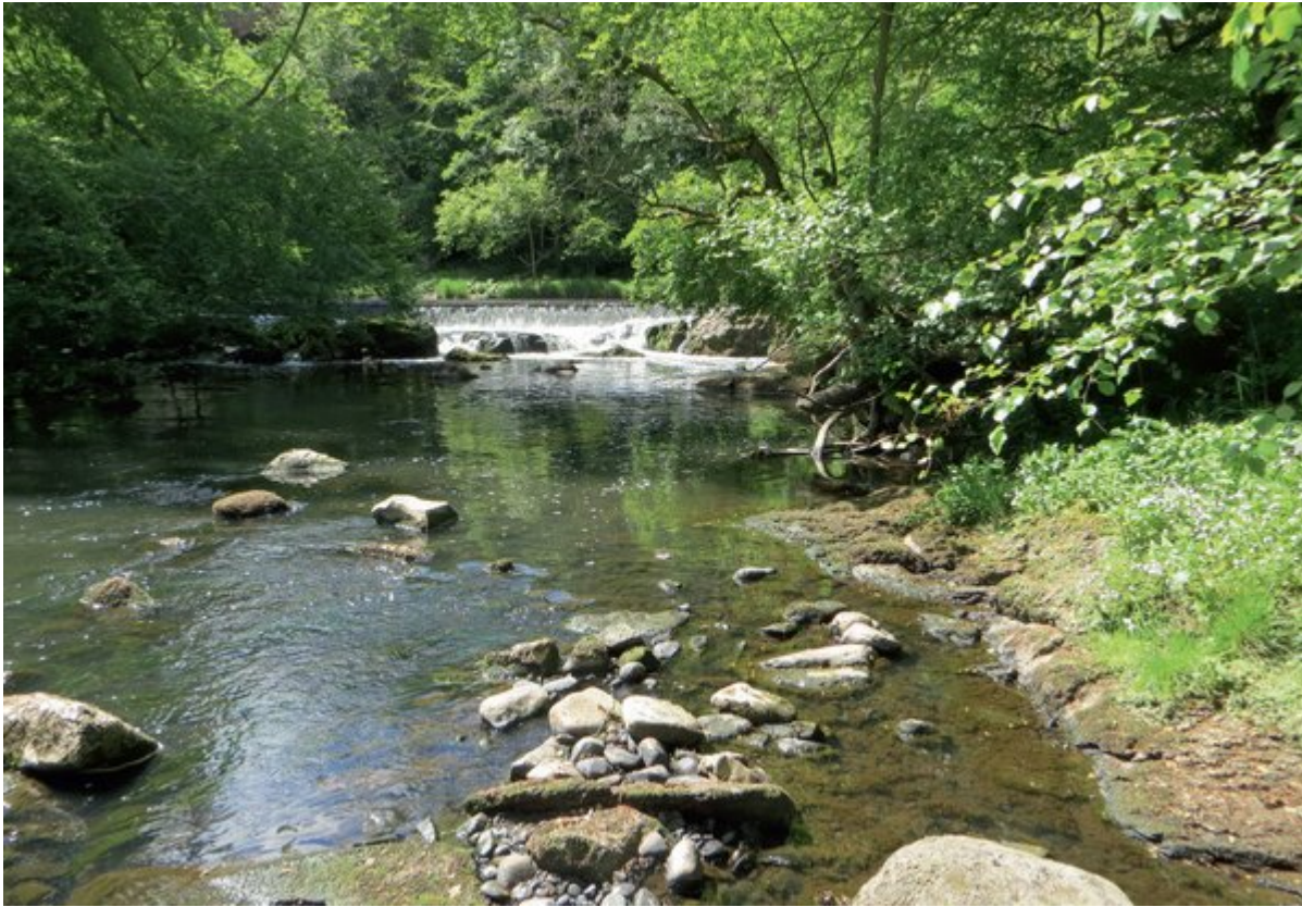
(Plate 4.3) Locality 4.6. Weir built on sandstone at base of Passage Formation above Castlecary Limestone, River Avon, downstream of Union Canal Aqueduct.
