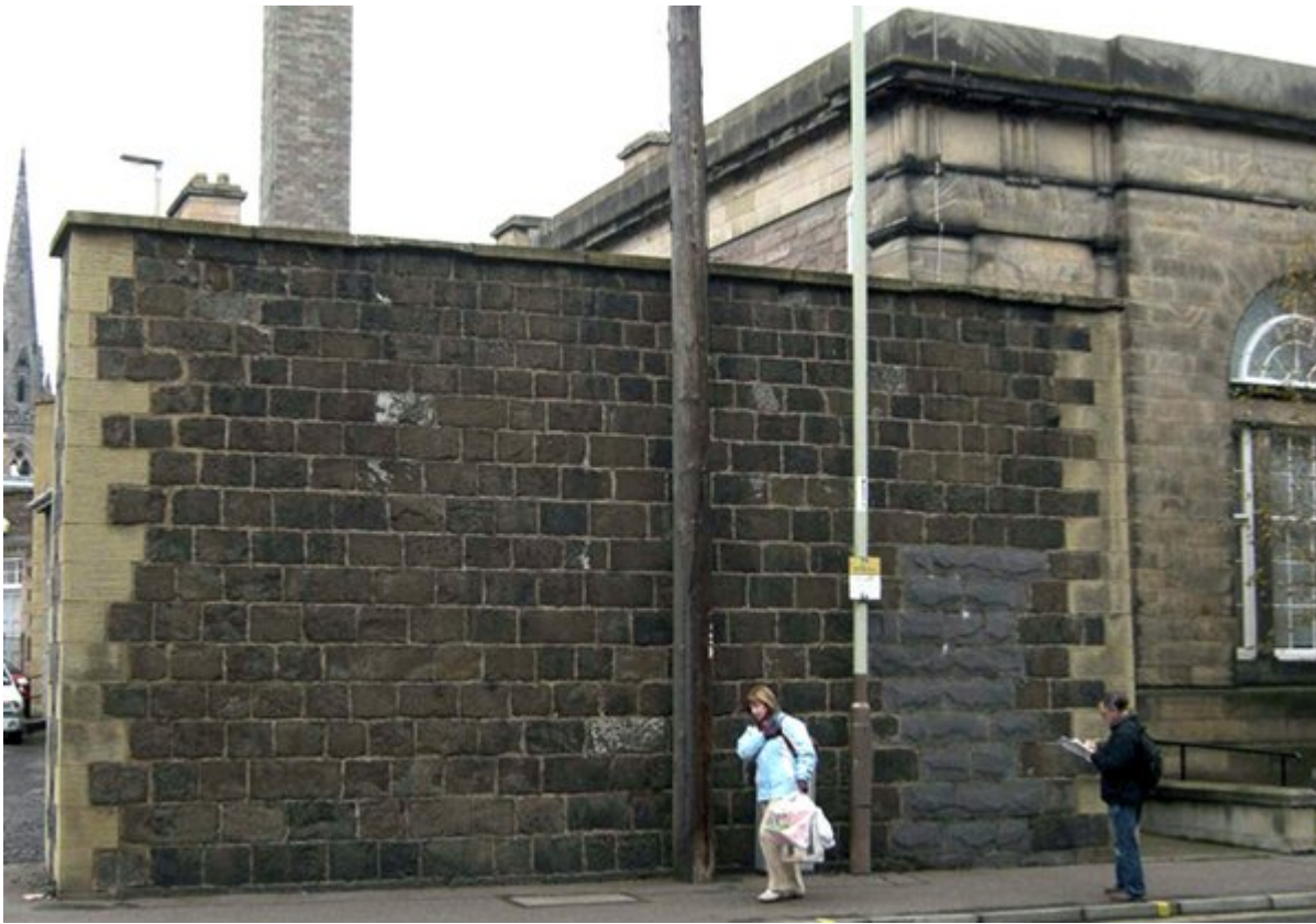
(Plate 16.4) Locality 16.11. Wall of demolished former town jail; quartz-dolerite from Lamberkine Quarry.
