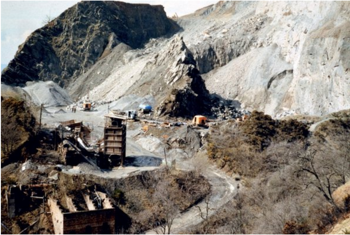
(Plate 7.1) Locality 7.4, Castle Craigs Quarry, Tillicoultry. Historic view towards the west of the quartz-dolerite (Midland Valley Sill-complex) in West Ochil Fault plane, with Ochil Volcanic Formation strata to right.
