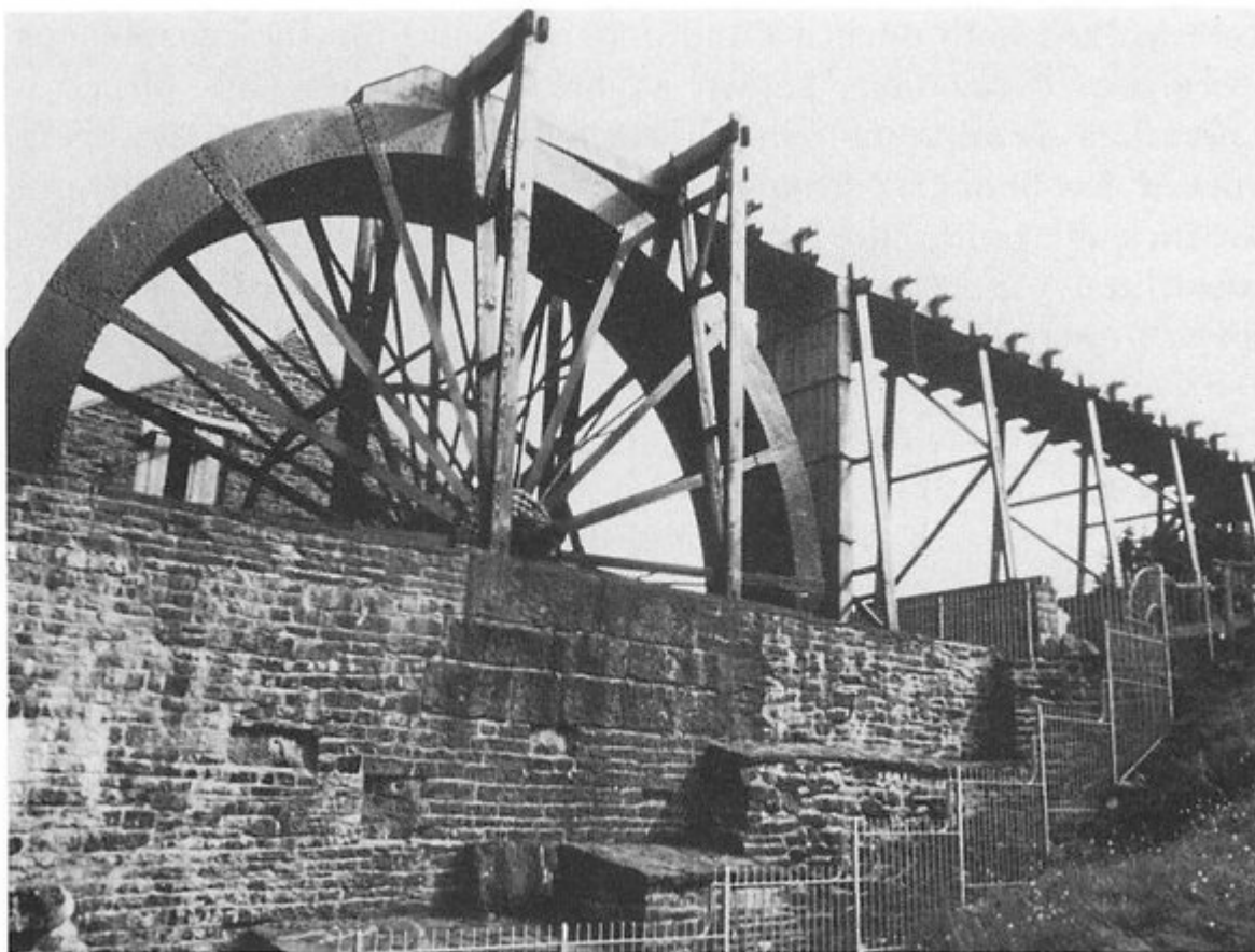
(Figure 14.2) Restored overshot wheel, Killhope Lead Mining Centre, Weardale. Photo: P. Nixon.
