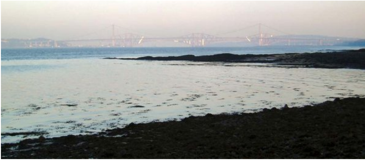
(Figure 60) The Forth Bridges from Abercorn Point (WLGS 18).
