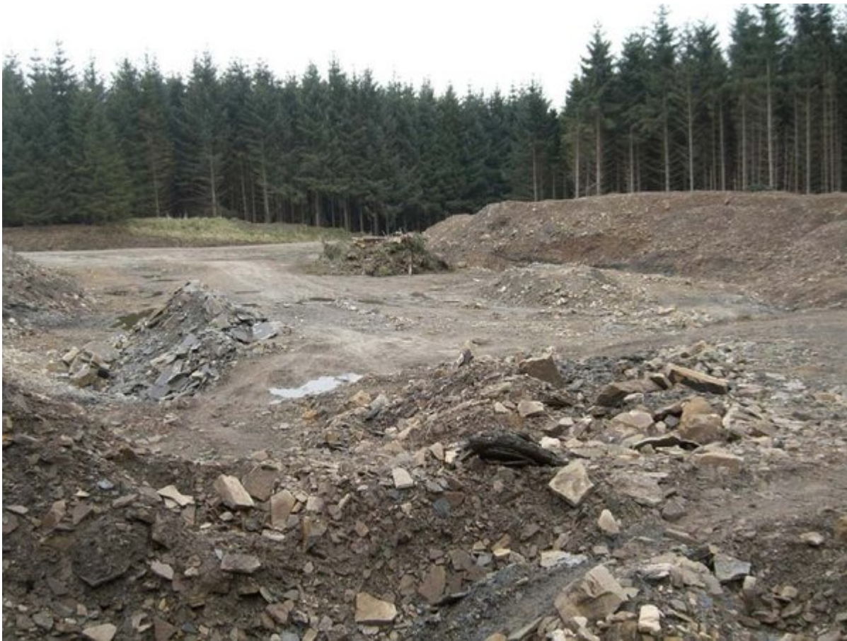
(Photo 207) Snatch quarry for track bases. The quarry is in sandstone with siltstone and mudstone beds belonging to the Lower Limestone Formation above the Blackhall Limestone. View looking southeast towards the small section displaying a fault.
