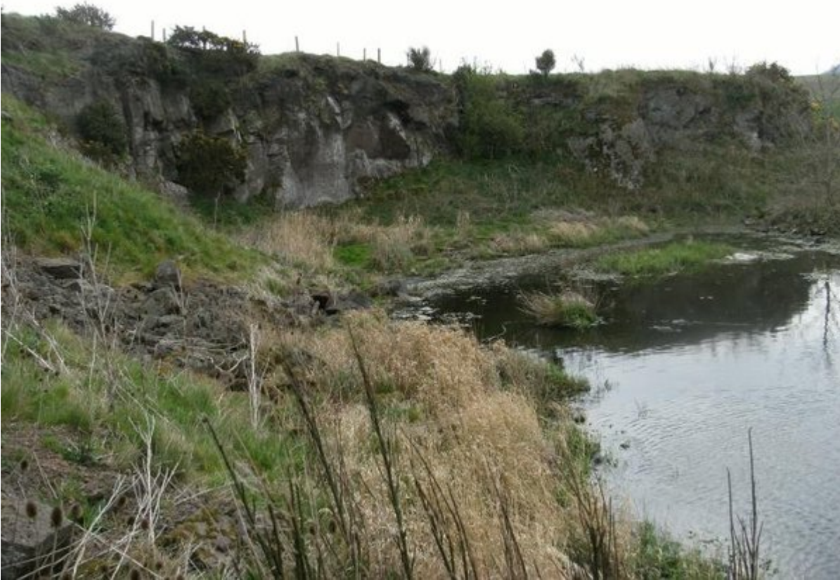
(ELC_7_P1) Overview of Old Markle Quarry. The floor of the quarry is filled with water, and the edges of the pond are littered with old bits of wood, rock debris, and other loose material. The accessible rock face is shown in this photo. Photo looking south. © BGS, NERC.
