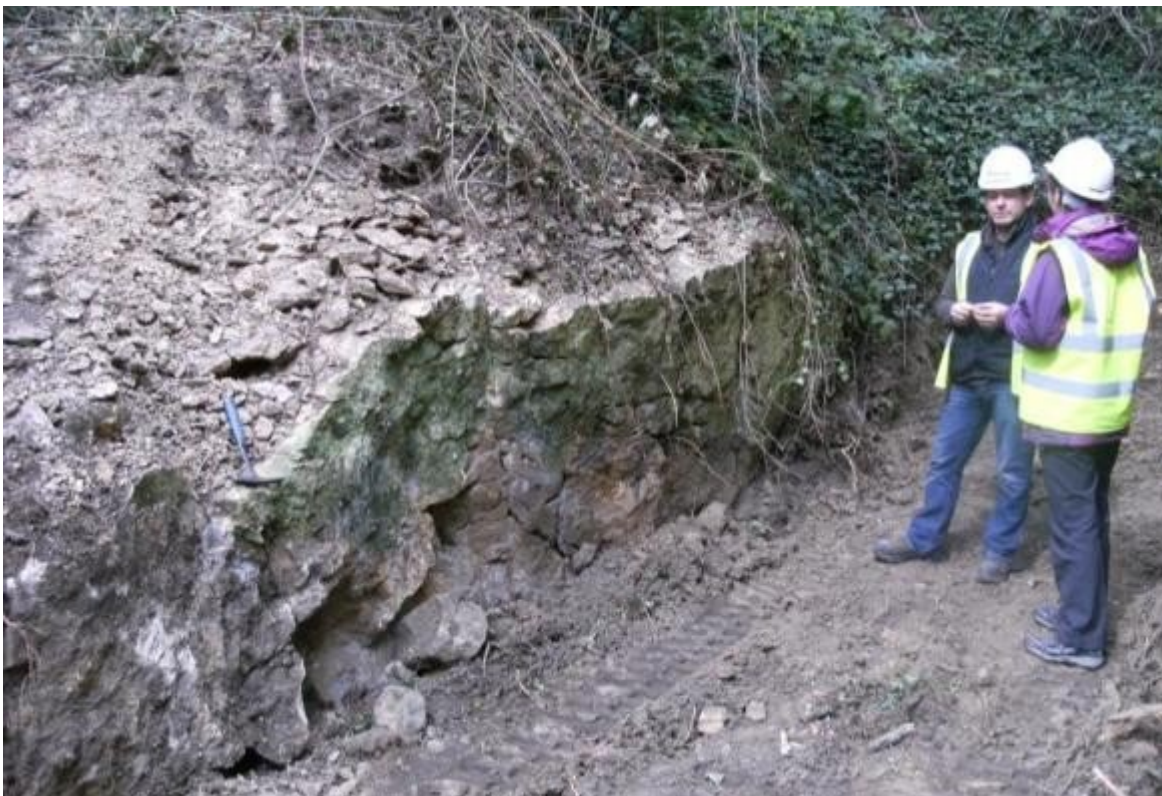
(ELC_12_P6) Ongoing work in the eastern part of the site has cleared material away the quarry face. Although the face will be left exposed, the floor is to be concreted and a fence constructed around the plot, impeding/preventing access to the exposure. Quarry face in the central part of the site. © BGS, NERC.
