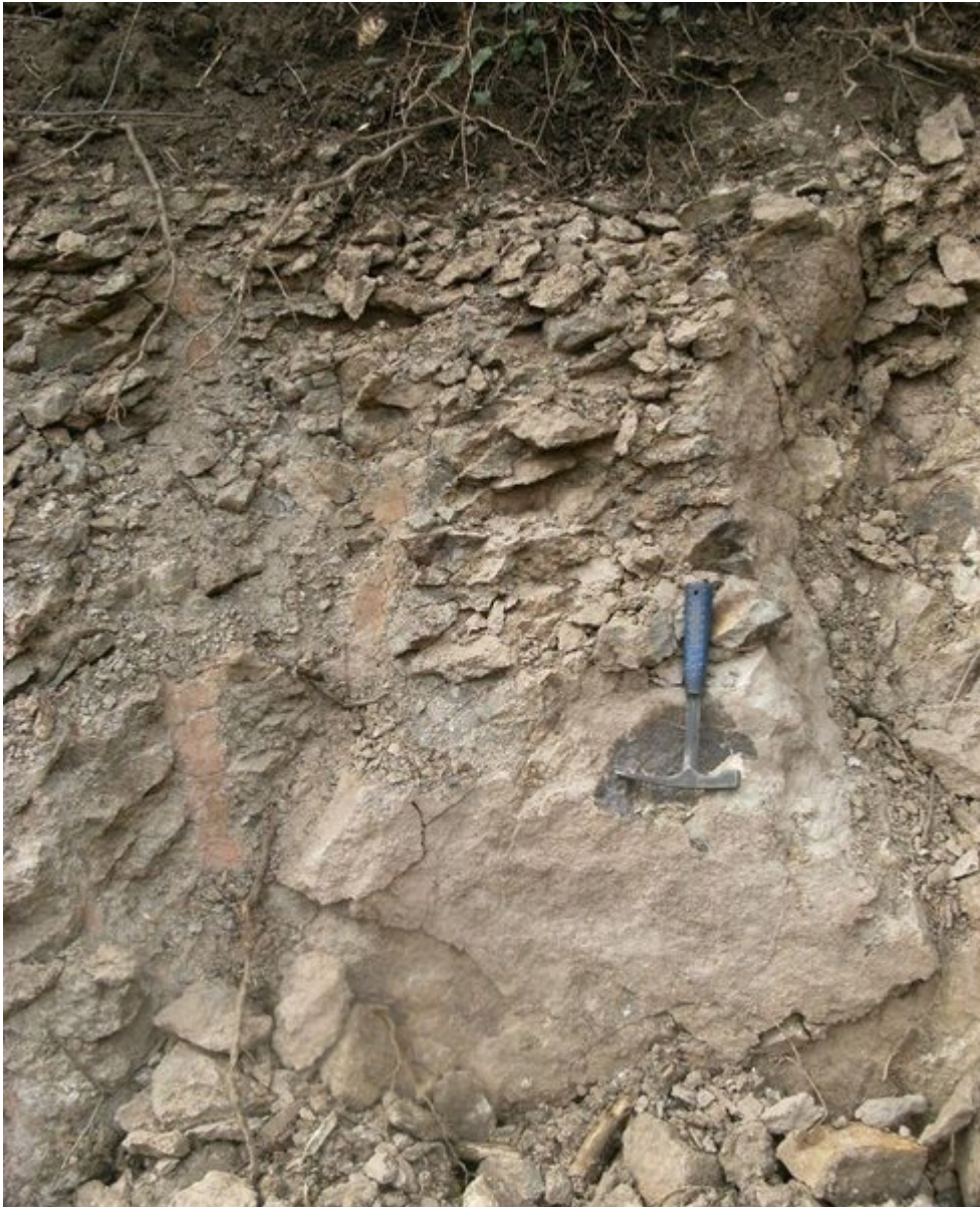
(ELC_12_P7) Detail of the uppermost part of the quarry face showing the increasingly weathered nature of the igneous rocks towards the natural surface. © BGS, NERC.
