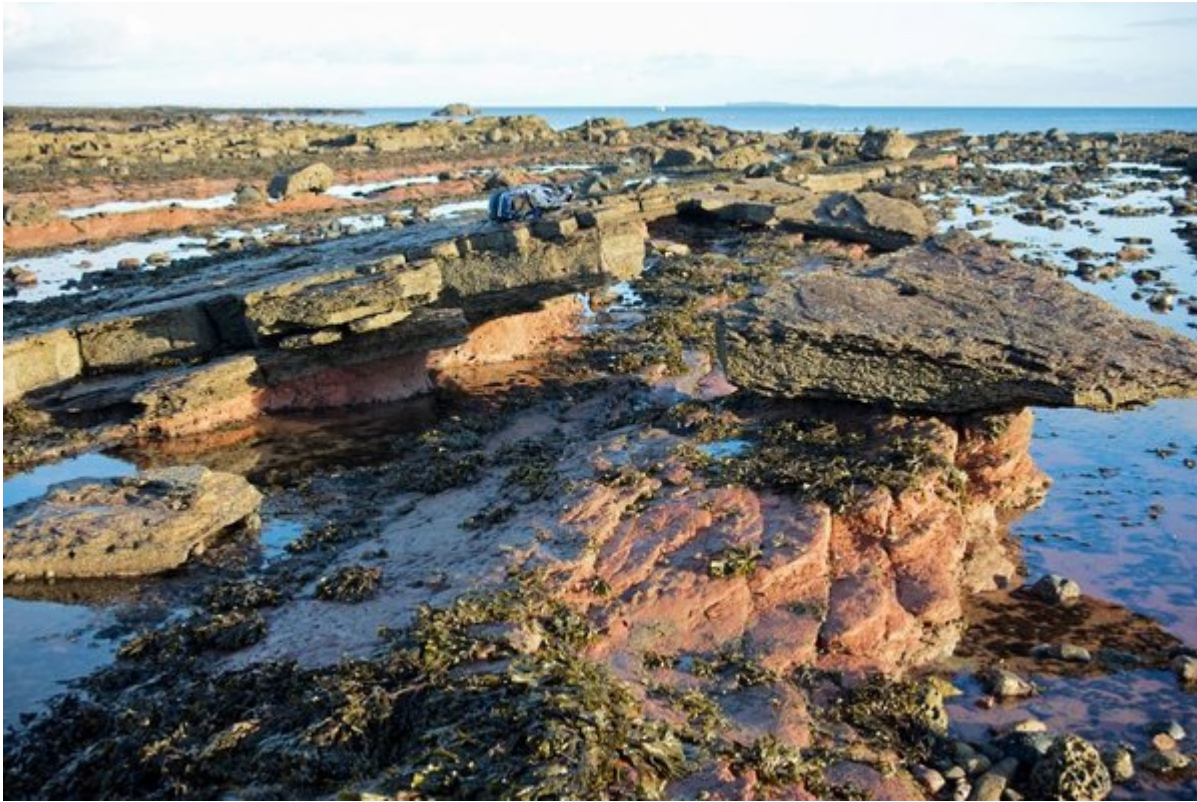
(ELC_25_P5) Undercut collapsed blocks on the shore platform south of Great Scar © John Gordon.
