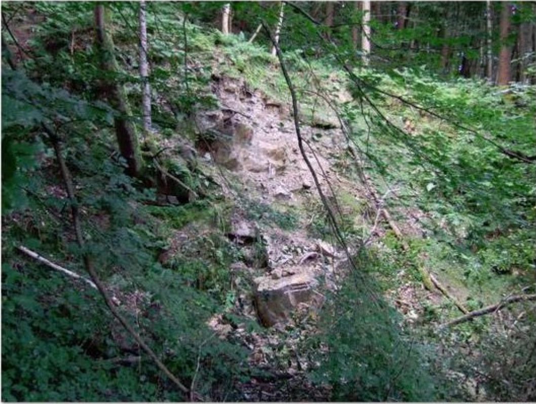
(Figure 15) SP 11. Rockfall. [NT 3728 5960]
