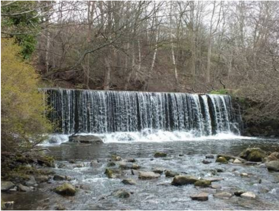
(Figure 23) SP 20. Weir, downstream from Catcune Mills. [NT 3502 6050]
