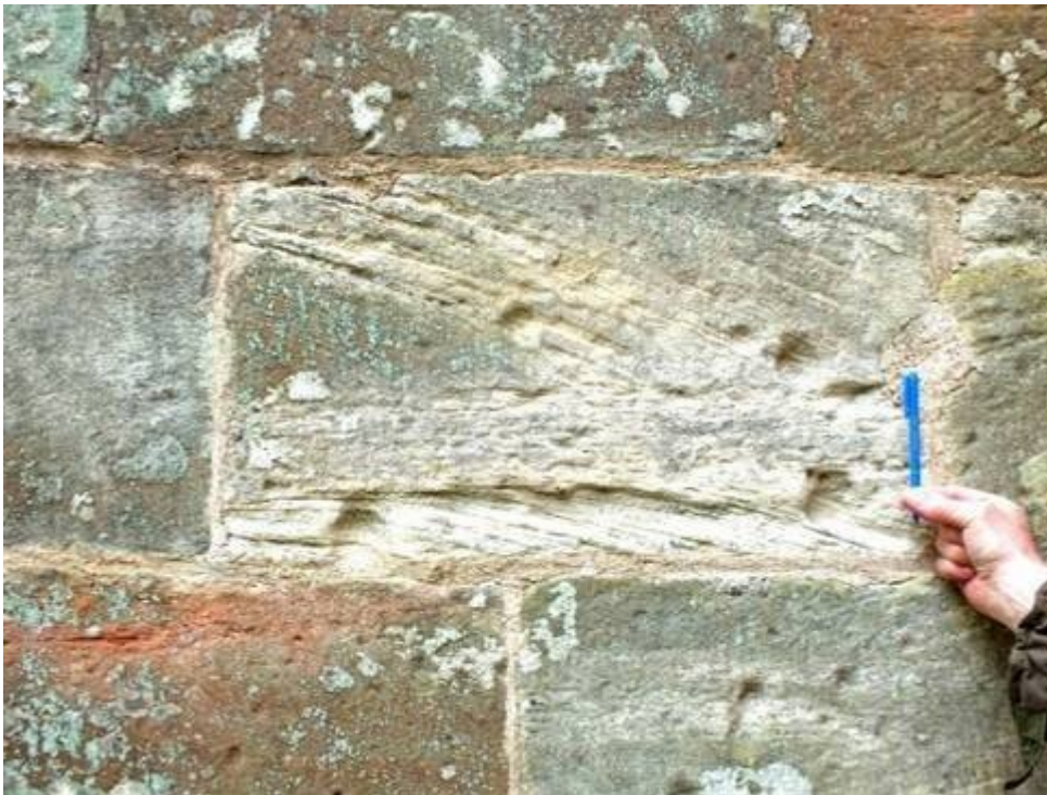
(Figure 6) SP 4. Crichton Kirk. [NT 3811 6161]. Geologically, this block is laid upside-down: the first layers deposited are at the top of the block, and were laid down at an angle. Then the tops of these layers were eroded before the second set of layers were laid down horizontally
