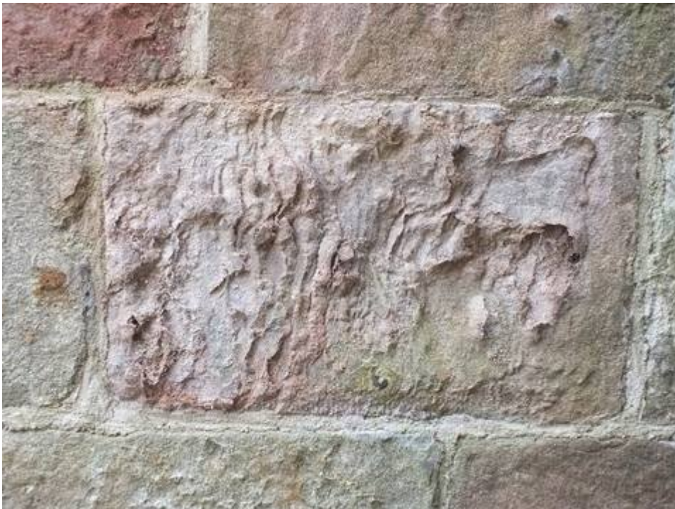
(Figure 8) SP 4. Crichton Kirk. [NT 3811 6161]. Cross bedding. Weathering has accentuated the features.
