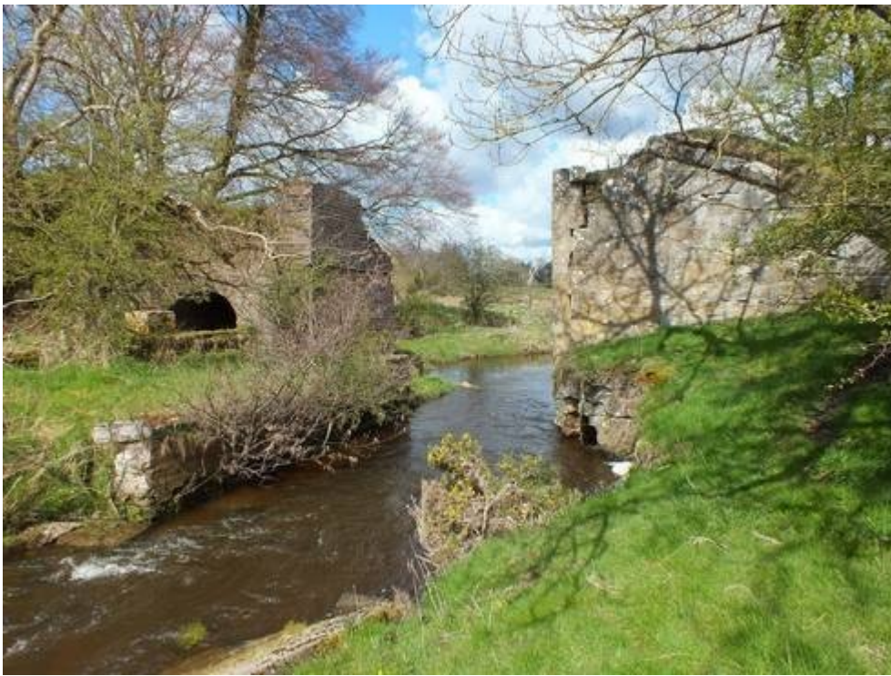
(Figure 19) SP 16. Broken Bridge. [NT 3539 5990].
