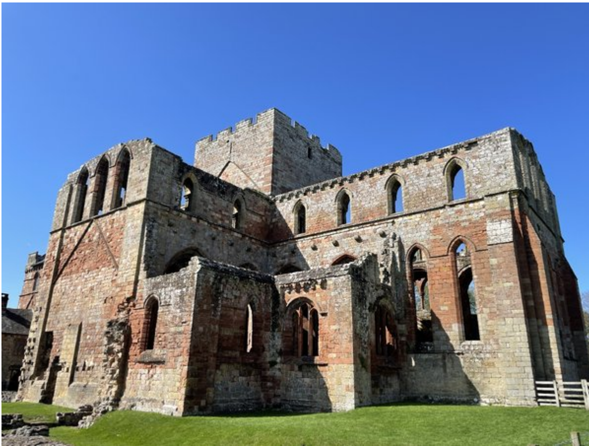
(Photo 11-1) Triassic and Carboniferous sandstone building stones in Lanercost Priory.
