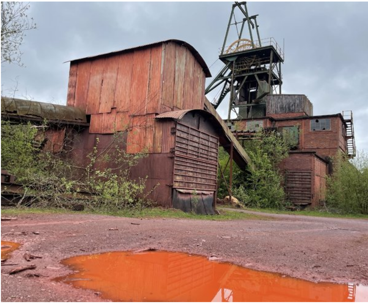
(Photo 46-1) Old buildings and shaft at Florence Mine.
