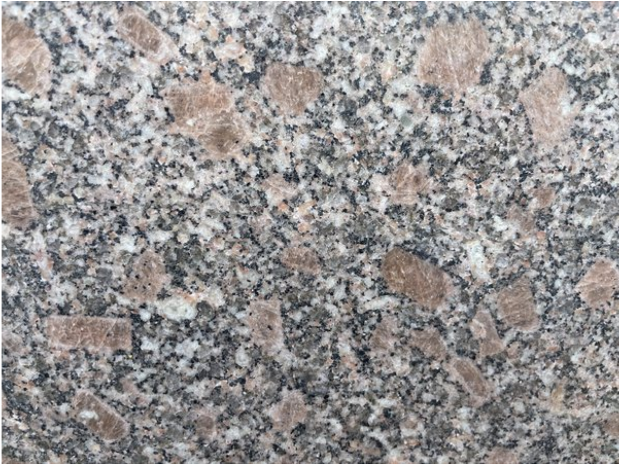
(Photo 21-2) Close-up of Shap granite.
