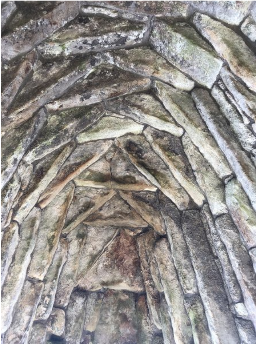
(Photo 00-3) Ceiling at Crindledykes limekiln.
