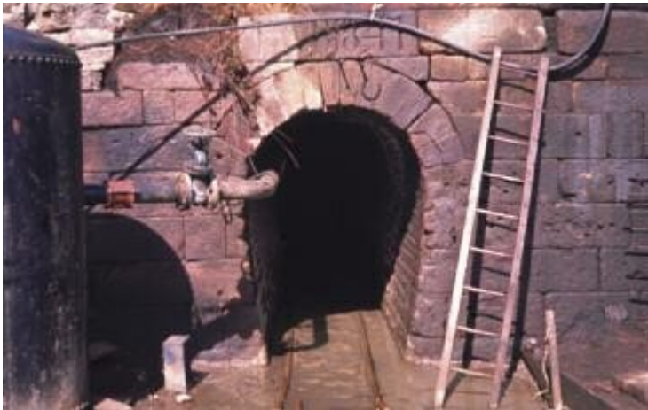
The original stone-arched entrance to Cambokeels Mine, Weardale, driven in the mid-19th Century. © B. Young, BGS, NERC.
