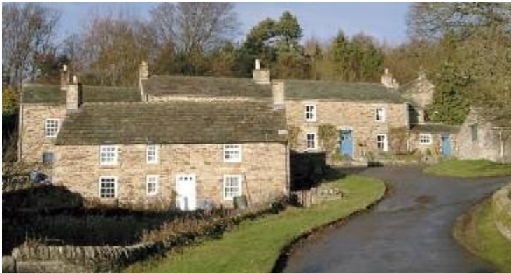
Blanchland – use of locally worked sandstones as building and roofing stone' © B. Young, BGS, NERC.
