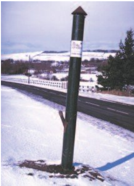
(Photo 21) Gas vent to allow drainage of mine gases from old workings. B Young, BGS, ©NERC, 2004.
