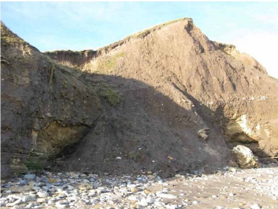
(Plate 12) Till (Boulder Clay) slippage in the cliffs north of Seaham (November 2008).
