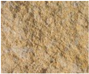
(Figure 80) The Inferior Oolite, known locally as Doulting Stone. [Inset].
