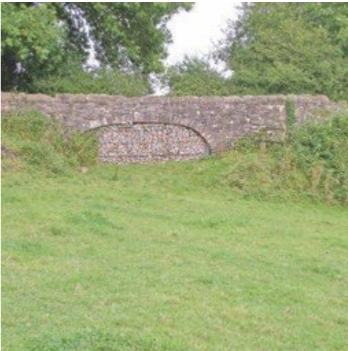
(Figure 58) Disused canal bridge, Edford.
