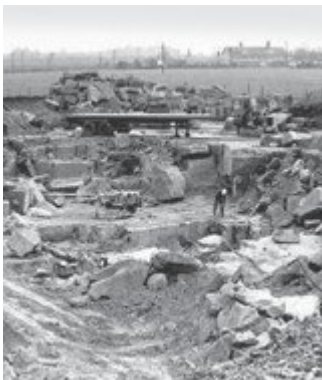
(Figure 76) Doultling Quarry in operation. Courtesy National Stone Centre, F Davies collection.
