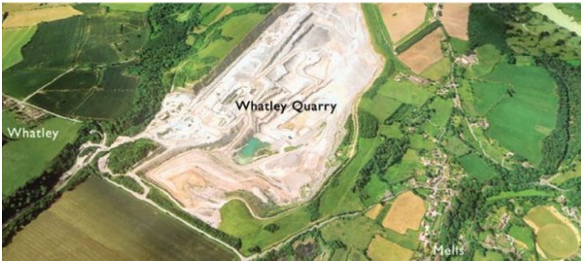
(Figure 28) Aerial photograph of the Mells and the Whatley area.
