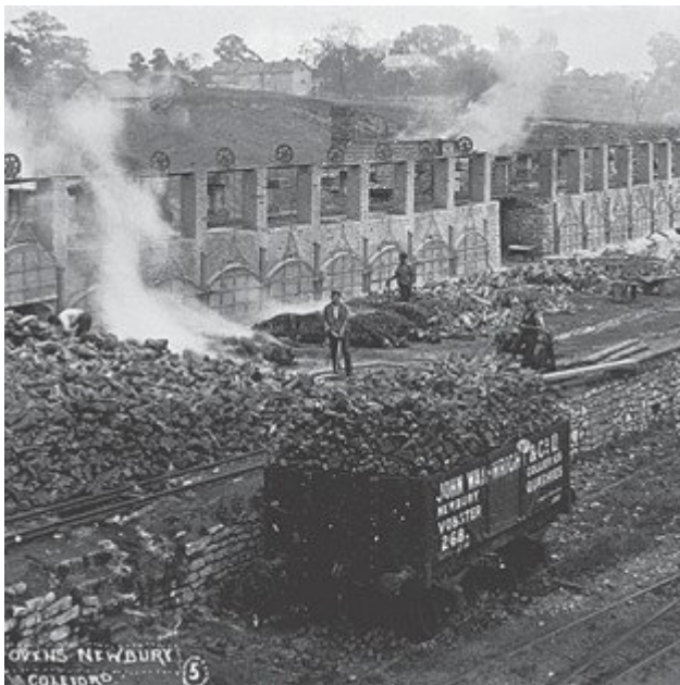
(Figure 36) Wainwright's Newbury Colliery showing the extensive coke ovens and some of Wainwright's privately owned rail wagons. Courtesy of the John Cornwell collection.
