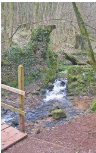
(Figure 106) Old mill waterworks, Harridge Wood.
