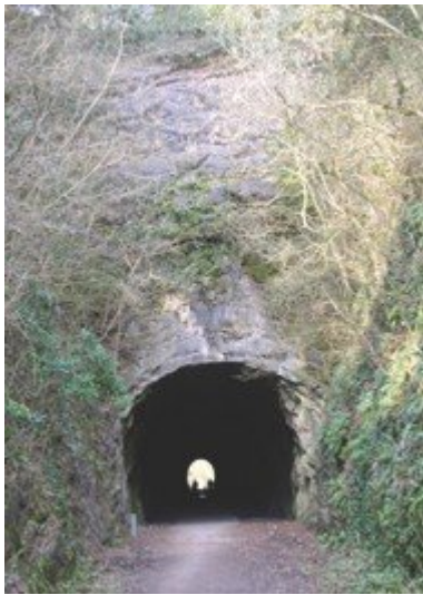
(Figure 67) Shute Shelve railway tunnel, a good exposure of the Black Rock Limestone on the cycle track between Axbridge and Winscombe.
