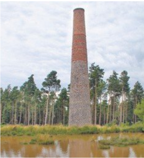
(Figure 113) Smitham Chimney, the last remaining lead-smelting chimney on Mendip, restored in the 1970s by the Mendip Society.
