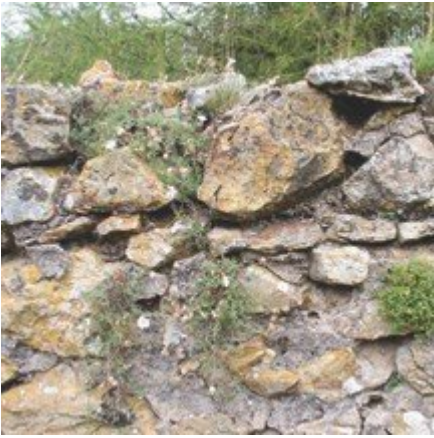
(Figure 112) The drystone walls on Smitham Hill contain large blocks of silicified Harptree Beds chert, with many lichens and small ferns thriving on the lime mortar.
