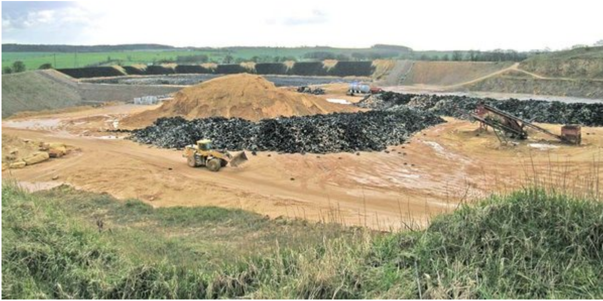
(Figure 41) General view to the south-west of landfill preparatory works. [SE 50063 11272].
