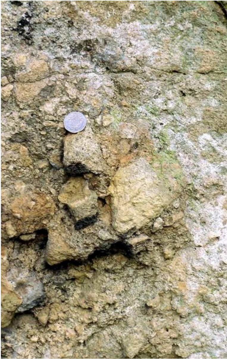
(Figure 55) Detail of limestone breccia along a joint running parallel to the quarry face. [SE 50868 01762].
