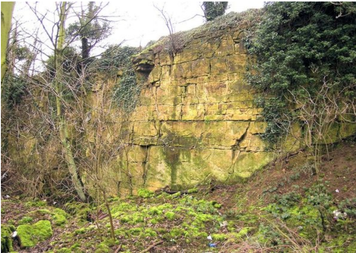
(Figure 80) Horizontal bedded limestones showing typical fracture patterns in the west quarry face. [SE 51487 12659].
