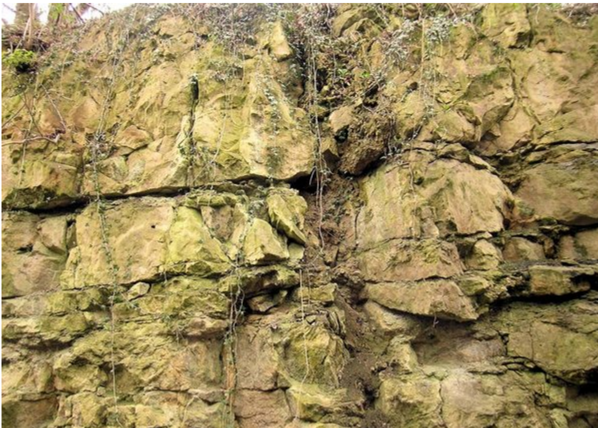
(Figure 86) A joint infilled with brecciated limestone fragments and unconsolidated Quaternary sandy clay. [SE 52750 00450].
