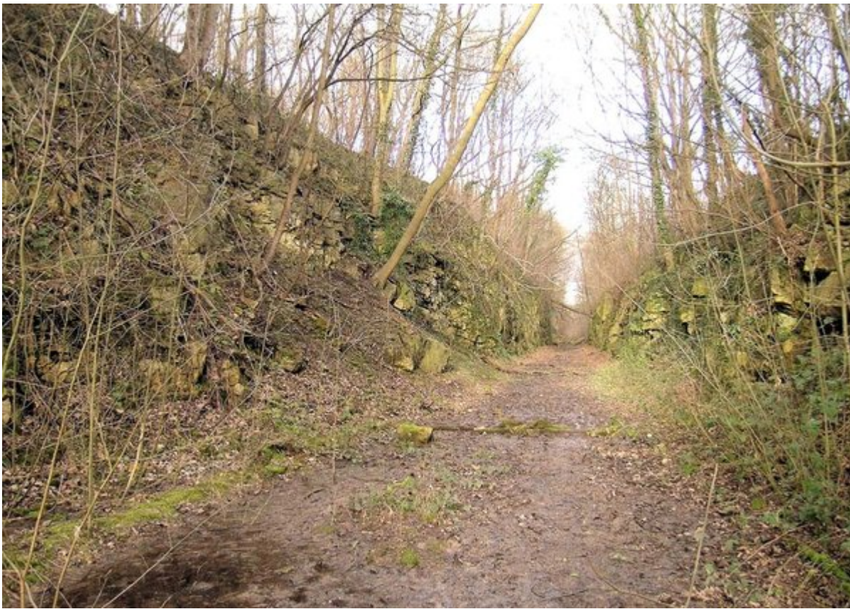
(Figure 83) General view east from centre of cutting. [SE 52785 00492].
