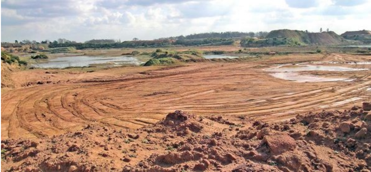
(Figure 142) General view to the west. [SE 65175 07905].
