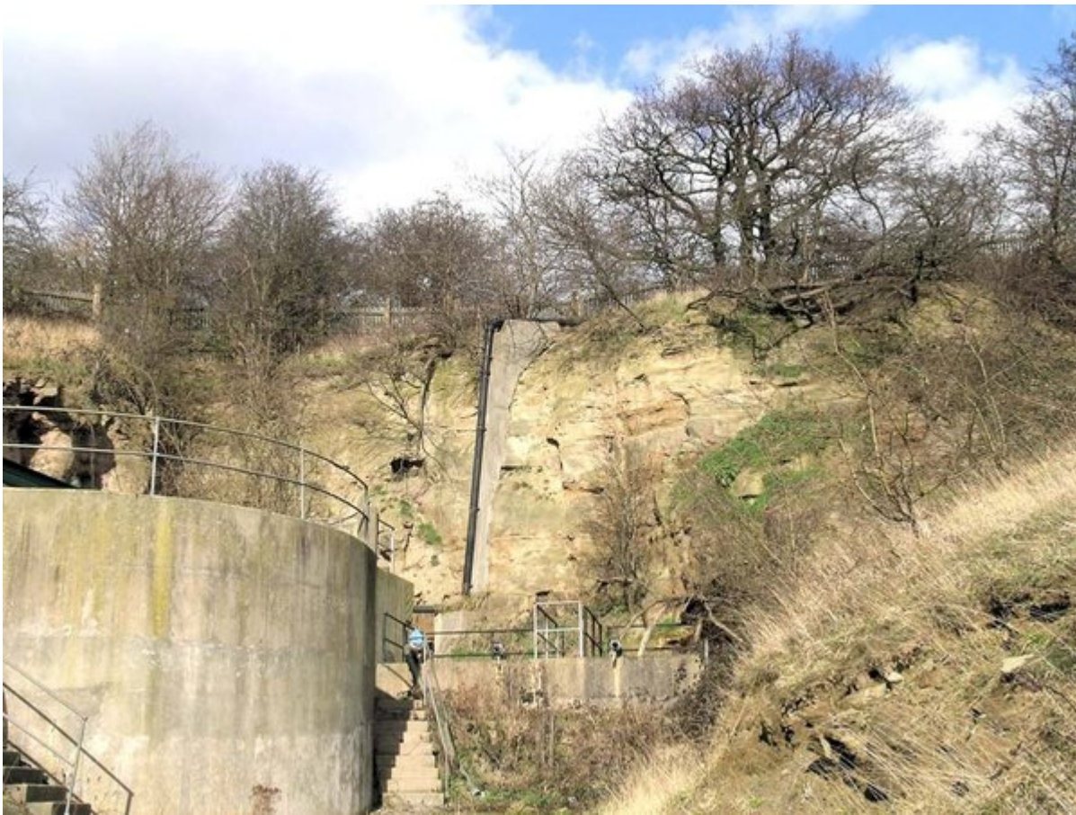
(Figure 28) General view of old quarry face. [SE 51205 00361].
