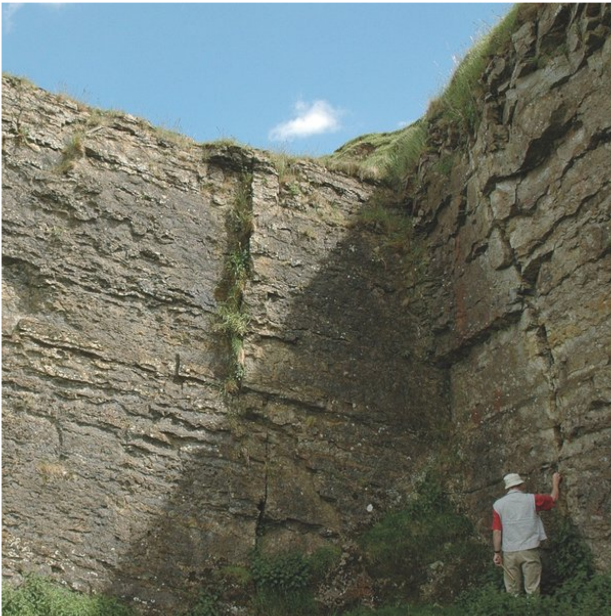
(Figure 30) Quarry in the Four Fathom Limestone near Milecastle Inn.
