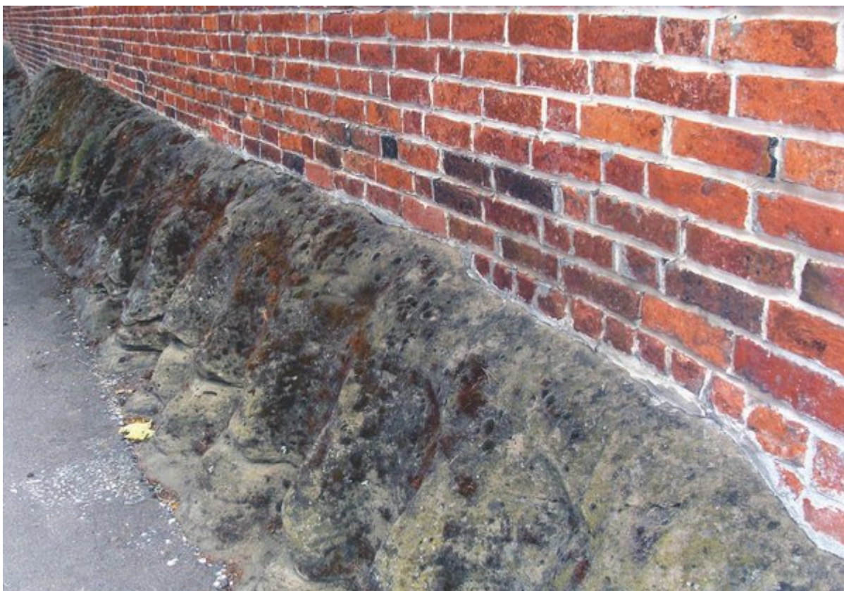
(Figure 58) Wall in Netherseal built on an outcrop of Bromsgrove Sandstone.
