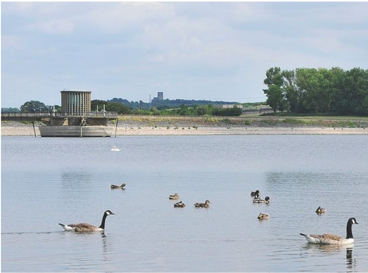
(Figure 75) Northern end of Staunton Harold reservoir.
