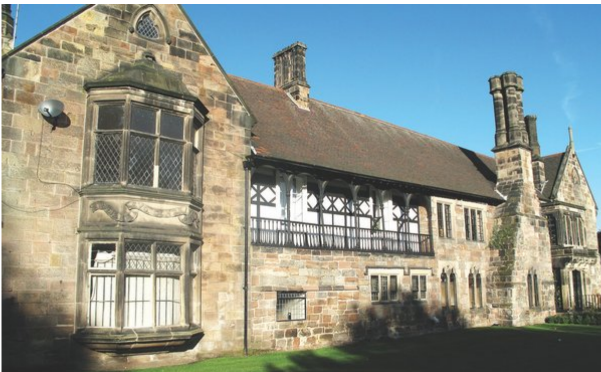
(Figure 105) The 'Abbey Inn' with its Triassic dressed sandstone stone blockwork. It contains part of the original Benedictine Burton Abbey Infirmary. It is on the river just south of the Market Hall.
