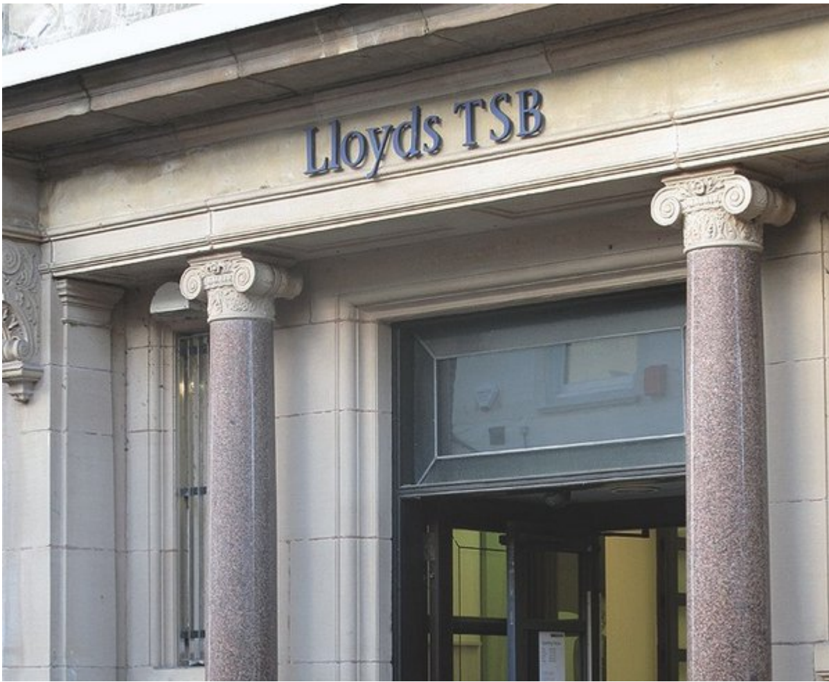
(Figure 101) Lloyds Bank building in Burton High Street. This is constructed using Millstone Grit sandstone but note the distinctive columns made of Scottish granite.
