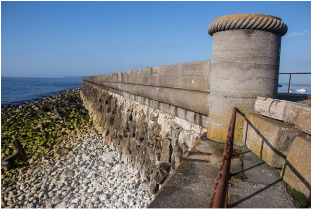
Dressed limestone blocks. Holyhead breakwater.
