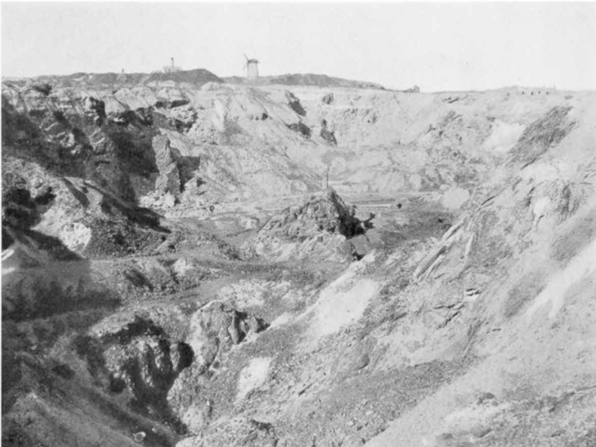
(Plate 60) Parys Mountain, the West Pit looking towards the summit. Silurian Shale, Silicified Shale, Felsite, Boulder-clay, and Spoil-banks.
