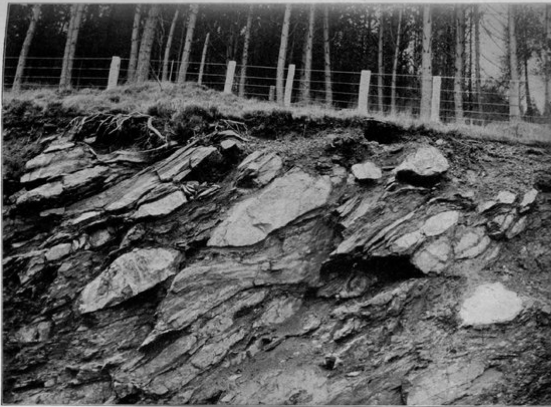
Phacoidal structure in Biotite-Gneiss and pegmatite, produced by post-Cambrian movements. Three-quarters of a mile west of Stromeferry Railway Station, Ross-shire.
