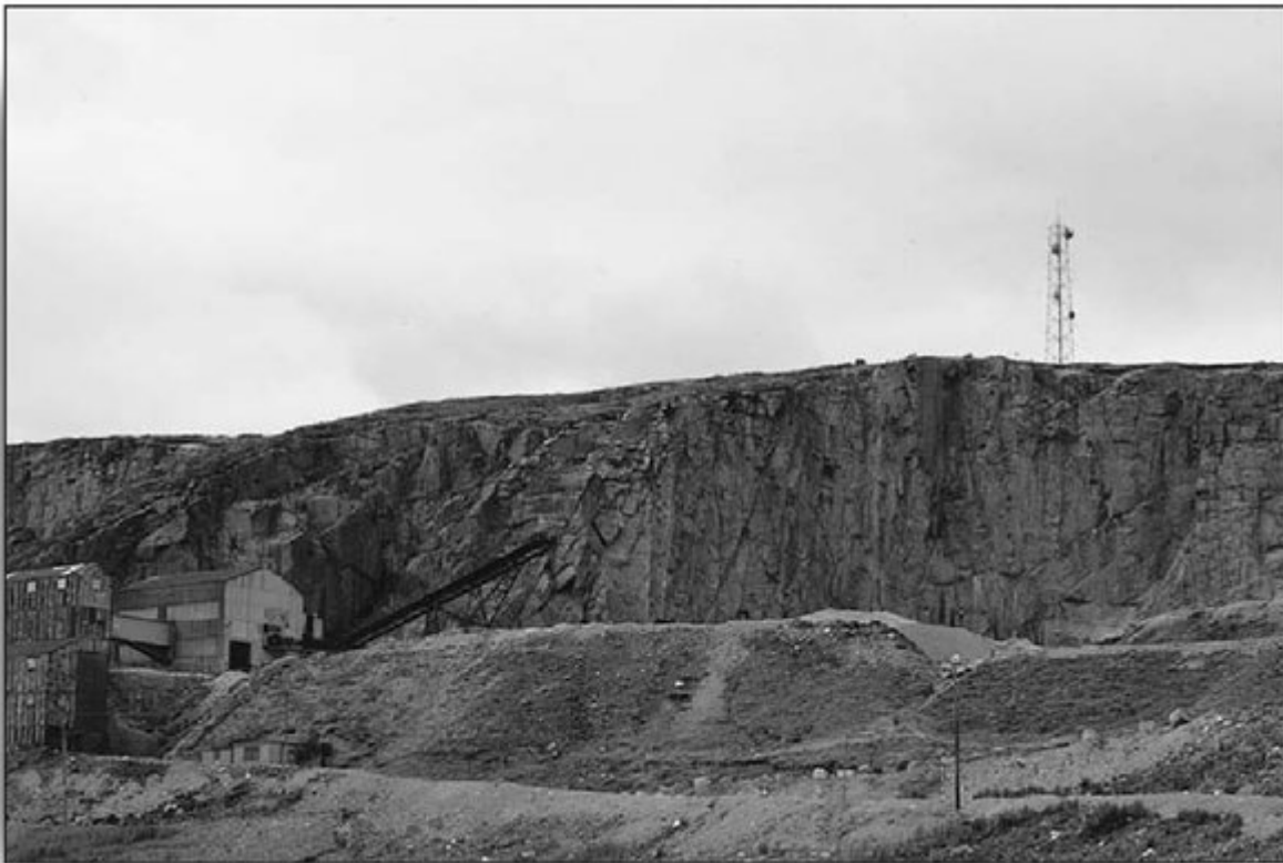
(Figure 67) The Shap Granite Quarry, Cumbria, showing regular jointing and the unstable face. This is an example of an exposure site. Photo: J.L. Evers.
